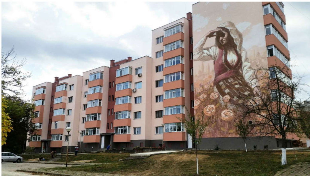
Figure 2. Example of a renovated building in the town of Smyadovo, Shumen Province, supported by the programme
