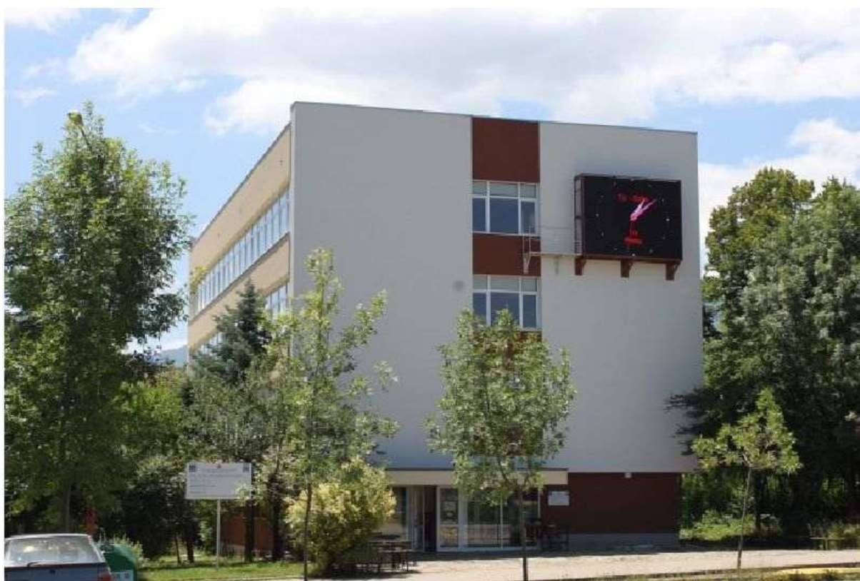
Figure 1. The first NZEB in Bulgaria, the Research Centre of the Technical University of Sofia.
